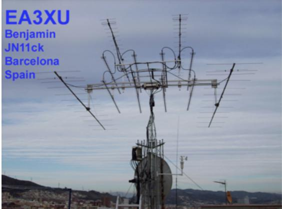
The serious antennas for the VHF/UHF and lower microwave bands, including 8 x 35 element yagis for 23cm consisting of two bayed boxes of four.
